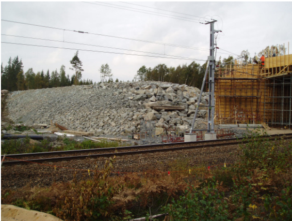
Pic. 4 - Build-up of embankment
