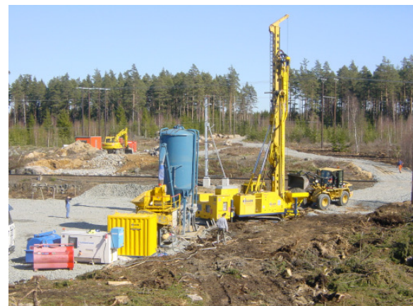
Pic. 2 - Site set-up
