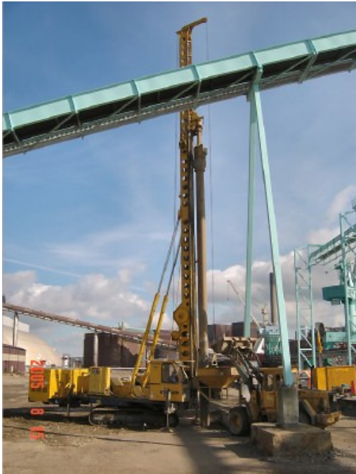
Pic. 5 - Site set-up
