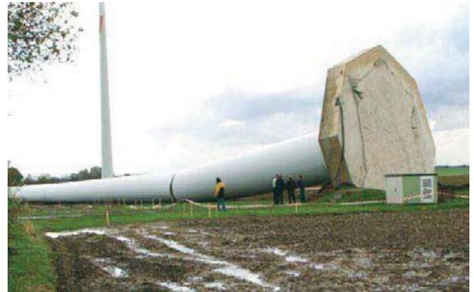
Figure 2. Overthrown wind energy plant in the wind farm Ellenstedt without soil improvement
