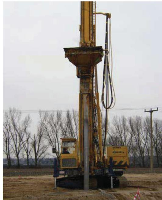
Figure 4. Compaction Example of construction of a Vibro Replacement Column
